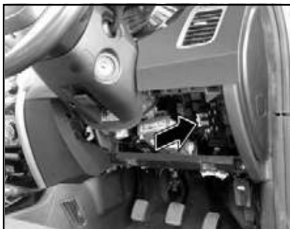
Fuse Box - Cabin Compartment
