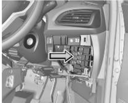
Cabin compartment fuse box
