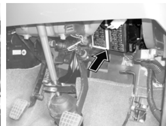
Fuses box in cabin (4SPTC) (Below dashboard)
