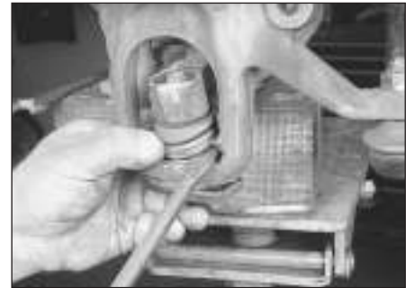
5.13 To detach the dust boot from the steering knuckle, pry the lower lip of the boot out of its groove in the knuckle
