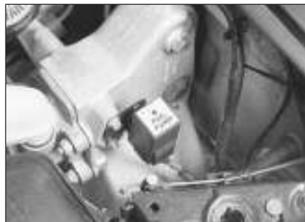
2.3c On 1992 models, the fuel pump relay is located in the left rear corner of the engine compartment
