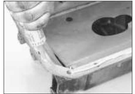
12.10 Apply a bead of RTV sealant around the perimeter of the sump mounting flange, be sure to run the bead around the outside all bolt the holes
