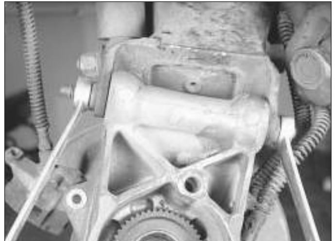
11.5 To detach the hub carrier from the rear control arm, remove the carrier-to-control arm nut and bolt
