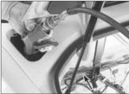
7.7b Direct low pressure compressed air into the hole for the overflow line if clogged
