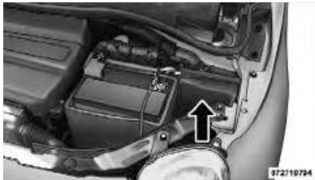
Front Distribution Unit
