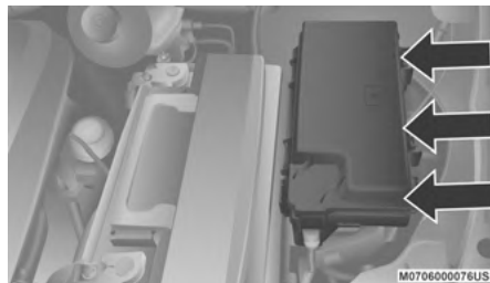
Totally Integrated Power Module
