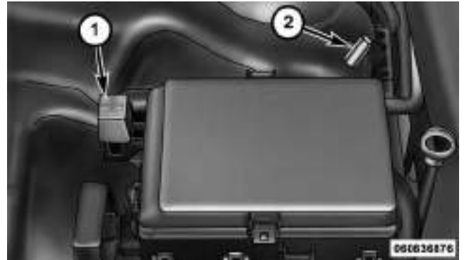
Remote Battery Posts Locations
