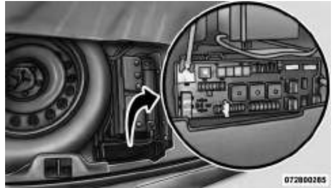
Rear Power Distribution Center
