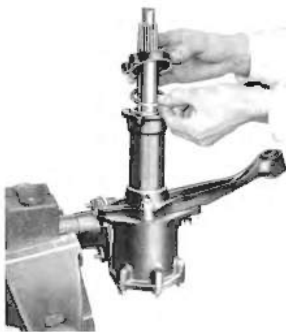
Fig. N20 Rocking shaft adjusting washer
