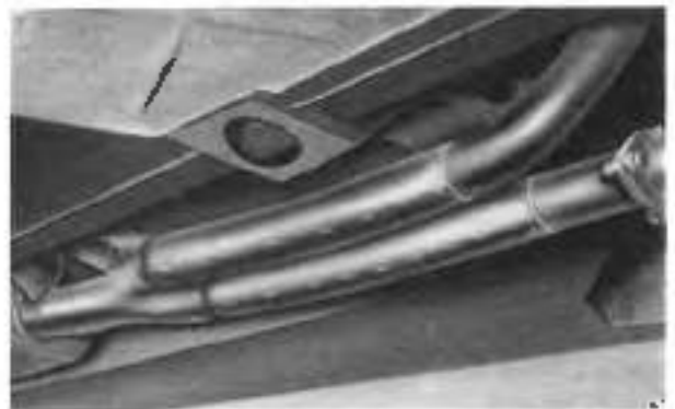
Fig. Q6 Position of exhaust pipe lagging
