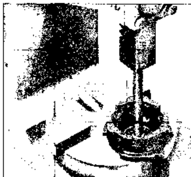
Fig. 5A-13 Removing Air Valve
