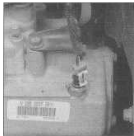
4.1 The back-up light switch is located on top of the transaxle case, near the left (driver's side) front corner
