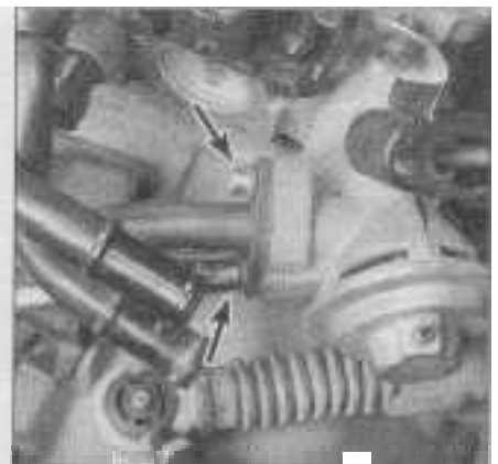
4.8 Remove the mounting bolts from the EGR tube (arrows) at the intake manifold and EGR valve (shown) and remove the tube
