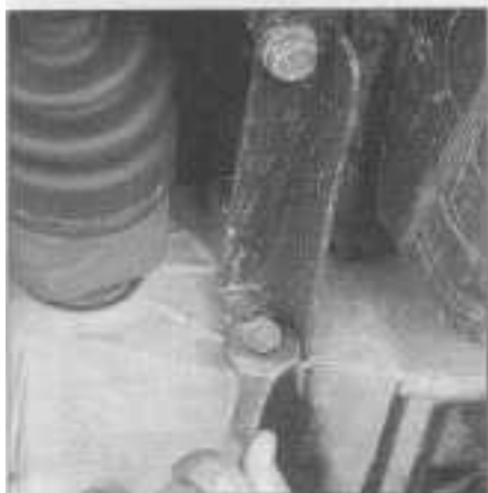
9.18 Removing a lateral strut bracket
