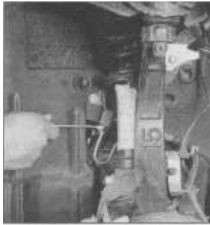
10.3 Disconnecting the front brake hose from the metal brake line using a flare-nut wrench
