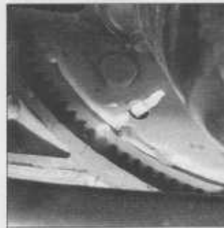
9.20 Before removing the driveplate-to-torque converter bolts, find a hole in the drive plate and match-mark the torque converter to the driveplate
