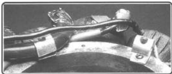
Figure 34. Fix for loose wiring.
