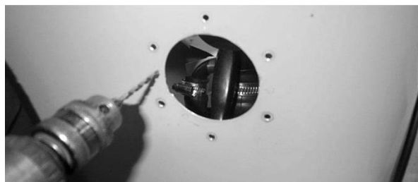
Figure 191: Carefully drill new holes
