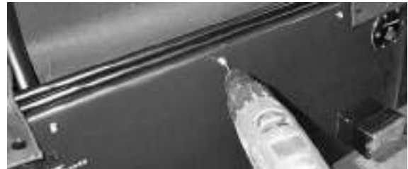
Figure 196: Drilling central popper on SV
