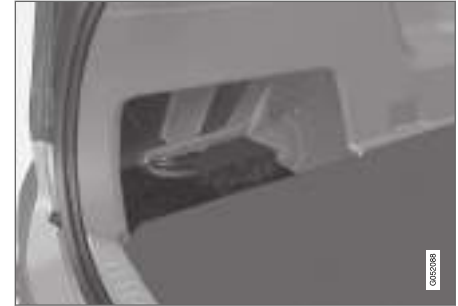
The starter battery is located in the cargo area.
