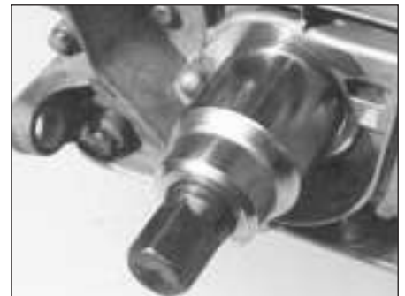
14.32 Using a large socket and the crankshaft pulley bolt to pull the oil seal into the housing (M40 engine)
