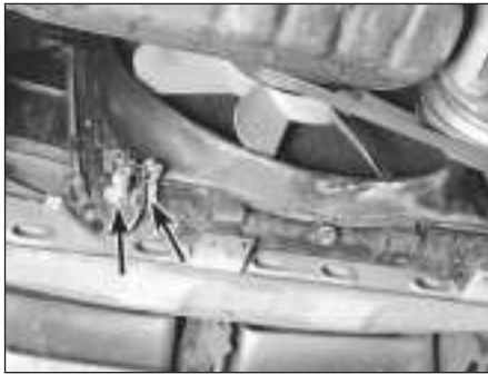
4.7 Sensors that control the high- and low-speed operation of the auxiliary cooling fan are located in various places in the radiator tanks
