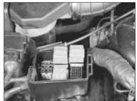
4.2 Engine compartment relays
